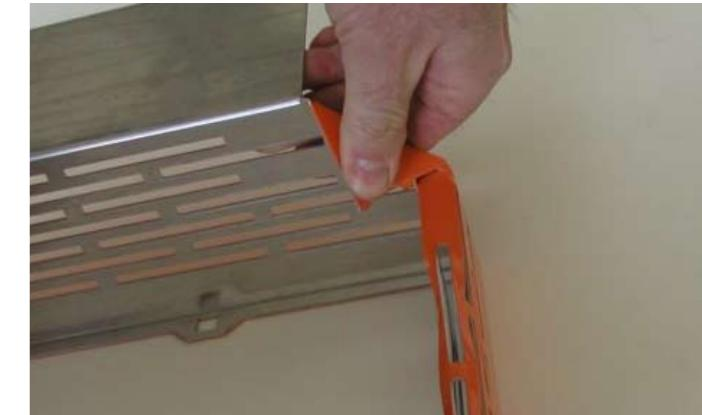
Cut away perforations (as shown) and bend tabs to allow clearance for angle fillets. Finally, fold rear panel (as shown) to clear the angle fillet and prevent exposure of any sharp edges.
